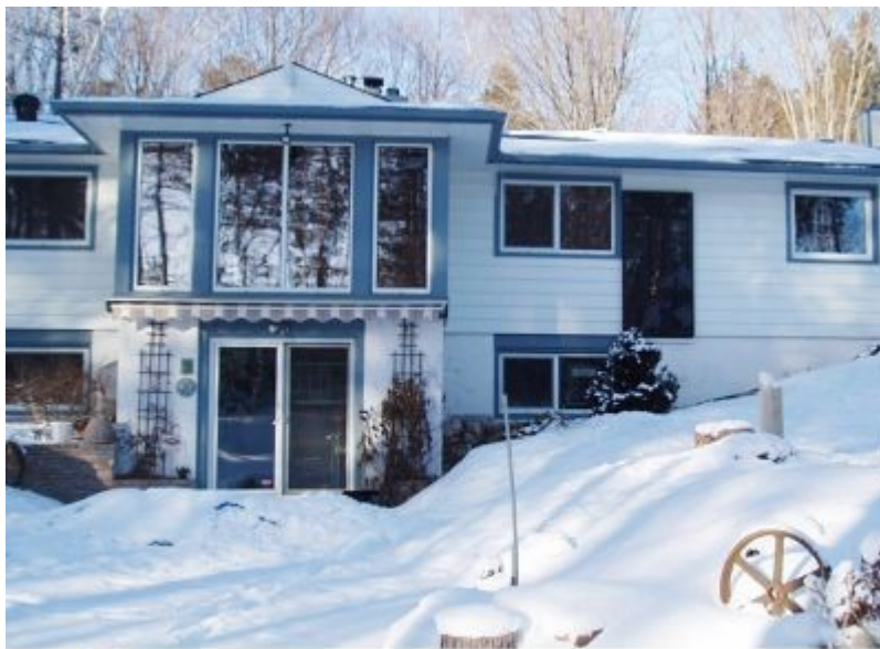
Enviro House with two wall integrated SolarSheat 1500G Solar Air Collectors Windsor, Ontario, Canada / Builder: BK Custom Homes
