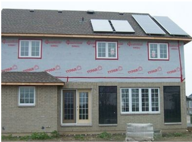
Enviro House with two wall integrated SolarSheat 1500G Solar Air Collectors Roof panels are Liquid Collectors and 1 kW PV system Windsor, Ontario, Canada / Builder: BK Custom Homes
