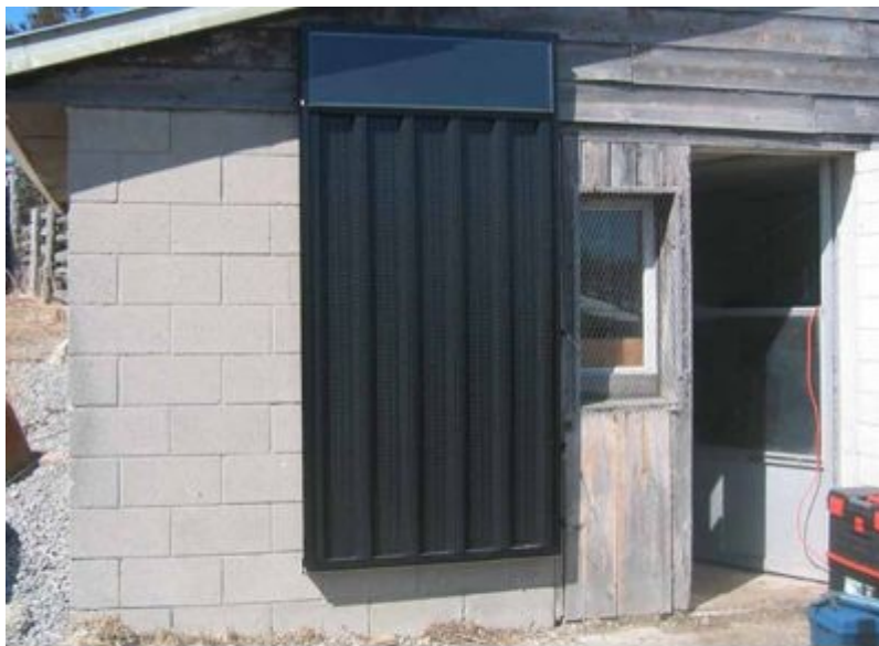
Enviro House with two wall integrated SolarSheat 1500G Solar Air Collectors Roof panels are Liquid Collectors and 1 kW PV system Windsor, Ontario, Canada / Builder: BK Custom Homes
