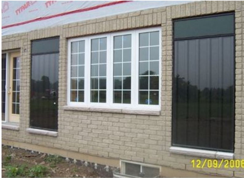
Enviro House with two wall integrated SolarSheat 1500G Solar Air Collectors Windsor, Ontario, Canada / Builder: BK Custom Homes
